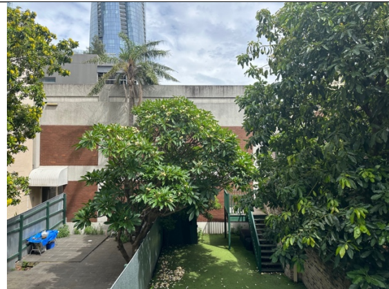
Figure 3.0, View from ground floor.
